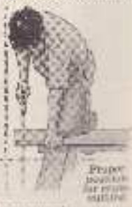
Proper position for ripping
